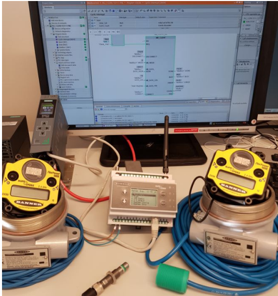
(a) PLC connected with computer and gateway
