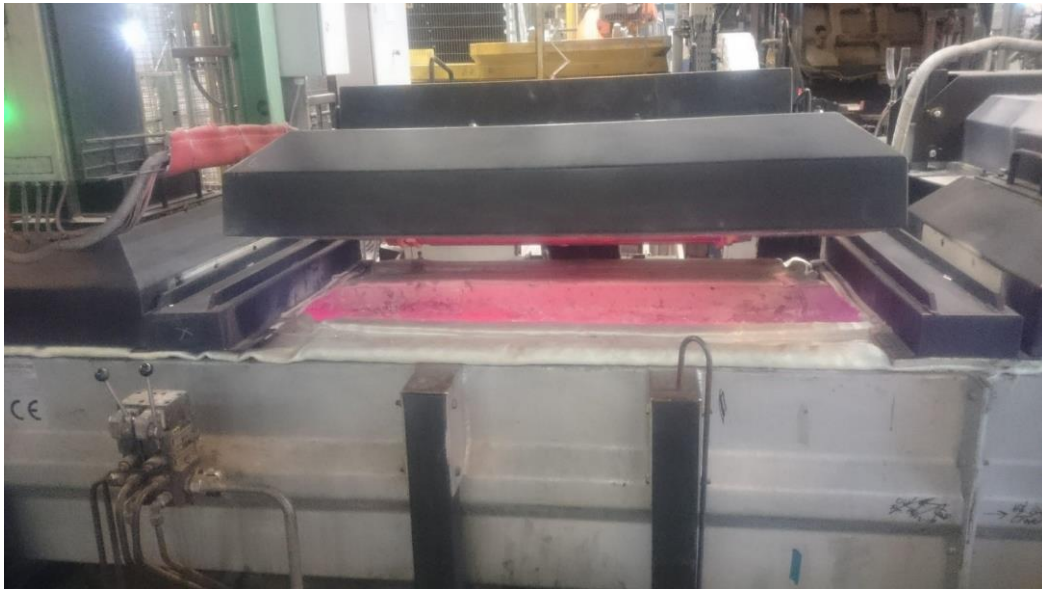
Figure 13: View of a chute carrying liquid aluminum
