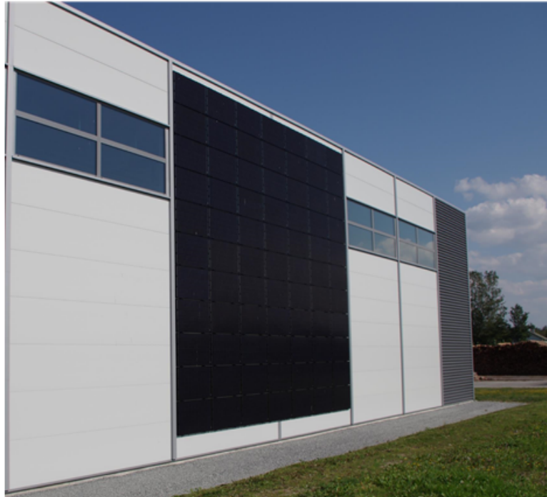
Figure 5.41: The BAPV system on the south facade of Haldenterminalen
