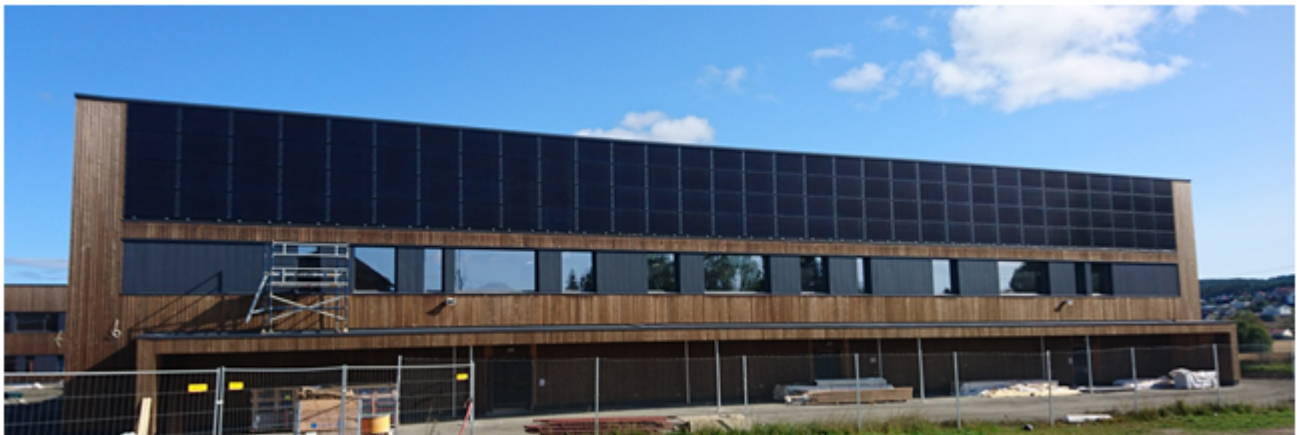
Figure 5.20: Picture of the south oriented BAPV at Bjørkelangen school
