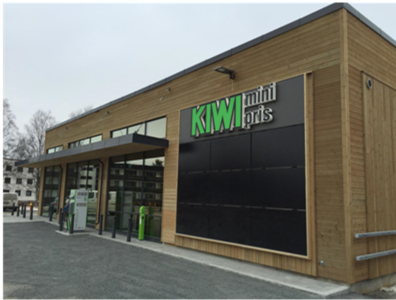
Figure 5.31: Picture of the south oriented BAPV facade at Kiwi Fjeldset, retrieved from [80]
