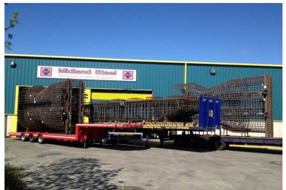
Figur 8-5: Ferdig armering transporteres [43].
