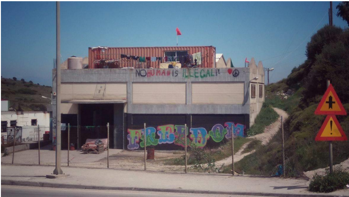
Figure 5: Outside NBK Warehouse (Source: Author).
