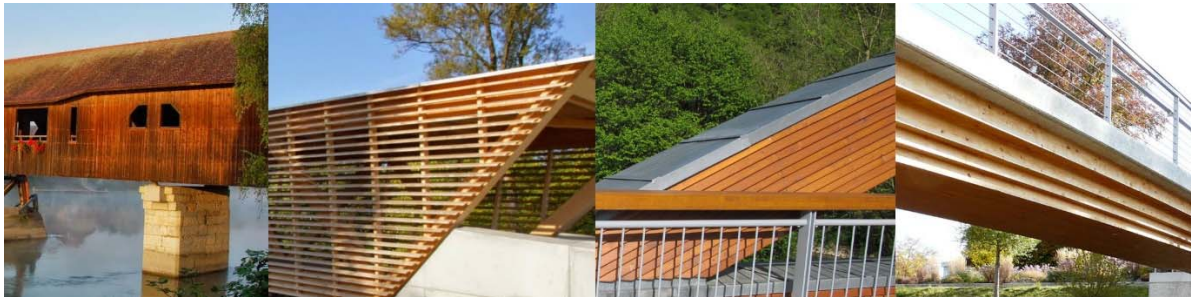
Fig. 1: Examples of structural protective measures – roof, housing, cladding, metal sheet, roof overhang and timber concrete composite structure
