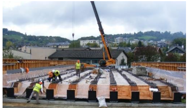
Fig. 25 Beams with metal plates for connection
