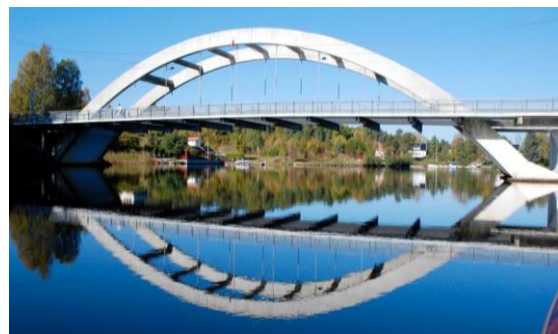
Figure 2. Existing Vippha Bridge [10]
