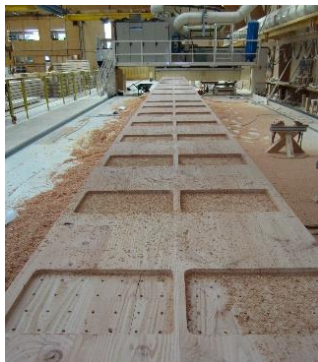
Fig. 21 Reserved spaces dug in beam
