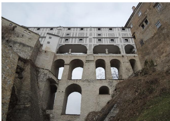
Fig. 4 The Cloak Bridge on stone piers
