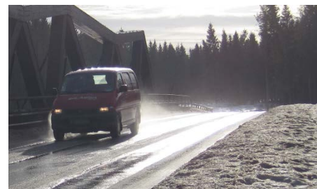
Figure 4 Standing water on bridge swirled up by each passing car
