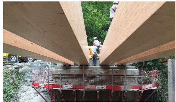
Fig. 20 View of the 4 girders
