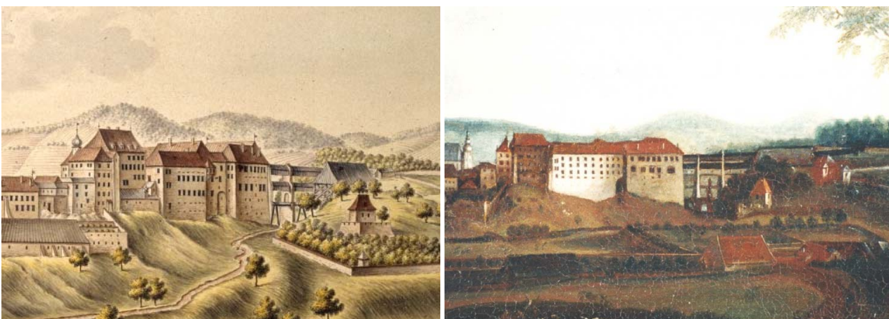
Fig. 4 Two views of the castle area from the north show the difference between the year 1724 (left) when the timber material of bridges and theatre building was apparent and after 1747 (right) when the lower corridor was widened and its wall cladding was plastered and painted.
