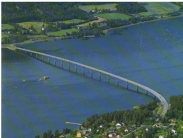
Figure 1 Overview of 1 st Mjøsa Bridge
