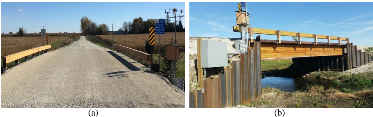
Fig. 1 August 2016 photographs of the completed Catt Bridge: (a) End view (b) Profile view
