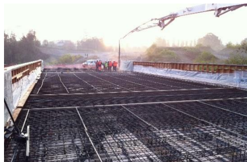
Fig. 27 Casting of the slab
