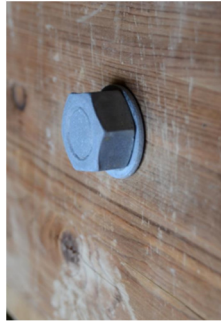
Loose bolts in girders and too small load distributing washers
