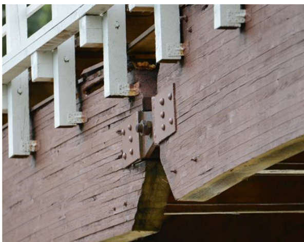
Deformation and decay in the top of the arch, the hinge is lost. Decay at the support of the arch.
