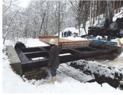
Fig. 12 Installation of CLT bridge decks
