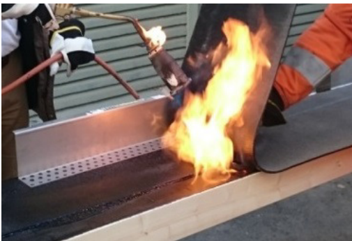
Fig. 6 Welding of waterproof bitumen sheet on edge steel angle
