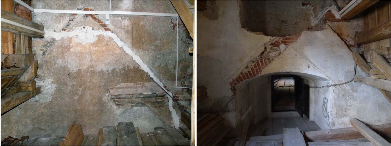
Fig. 6 The imprints of pitched roofs from both previous construction phases are still clearly recognizable. The best situation has survived on the outside wall of the castle palace (left) and on the exterior plaster of one of the brick pillars (right).
