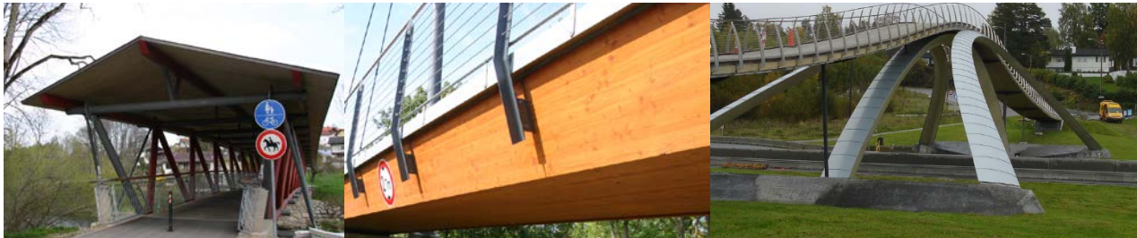
Figure 9 Example of modern bridges with inverted pyramid design. From left Traunreut, Taubersbischofsheim and Leonardo da Vinci bridge
