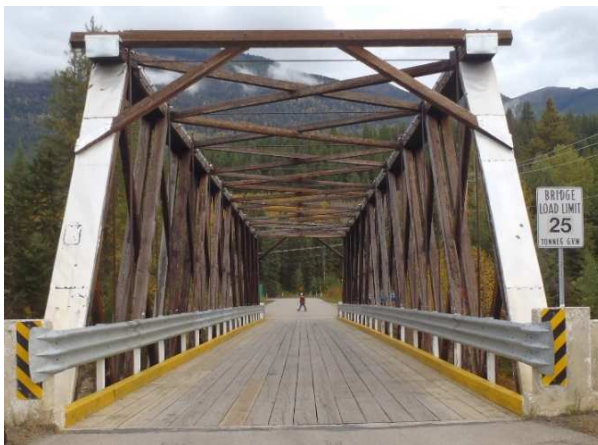
Fig. 8 Typical View on Deck, Through-Truss With Portal Bracing
