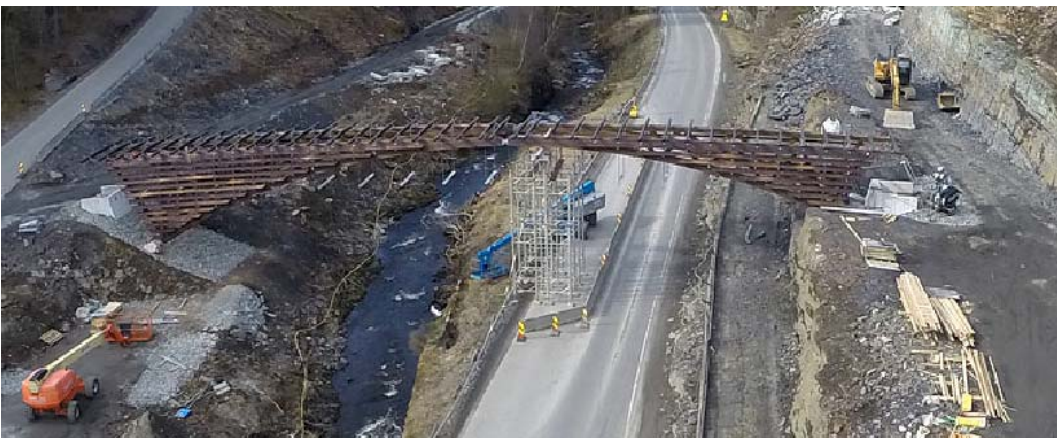
Figure 8 Construction of Bjørgum bridge seen from the air. Photo S. Ulvund
