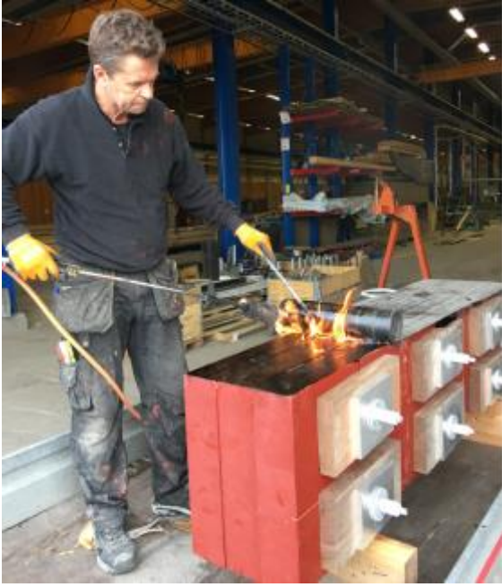
Fig. 4 attaching water proof membrane.
