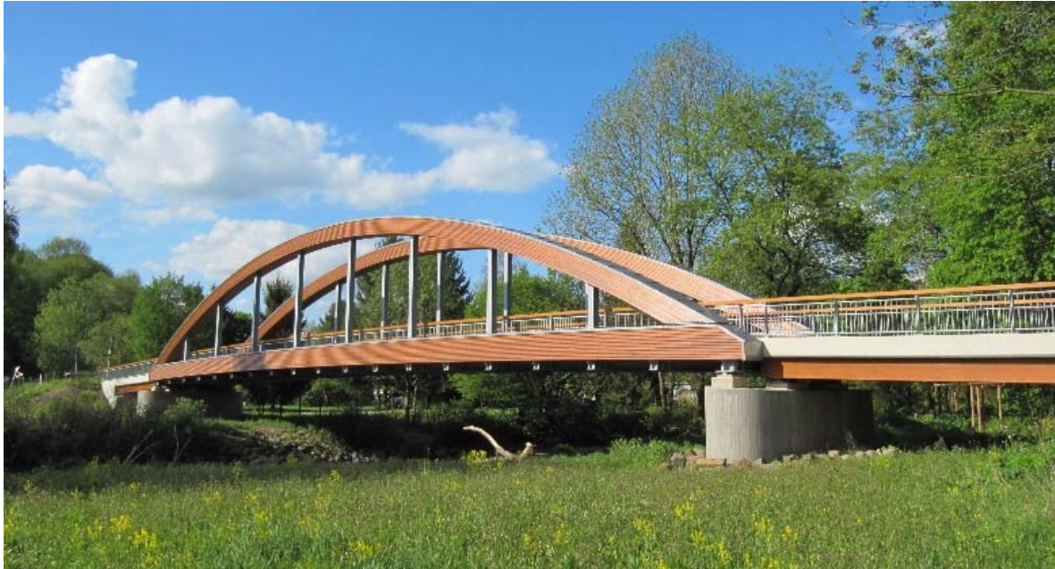
Fig. 4: Road bridge in Höngesberg
