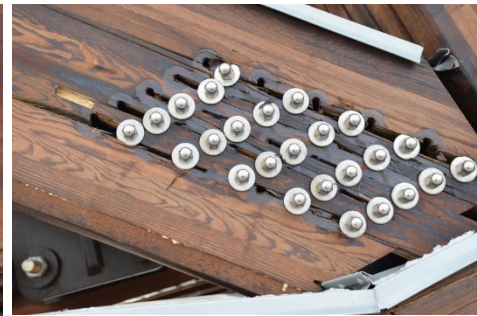
Figure 4 Example of group tear failure (left) and row shear failure (upper) on Perkolo Bridge
