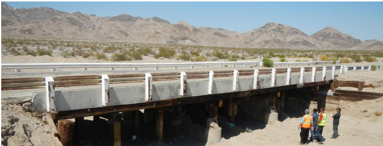
Fig. 3 TCC bridge along US Route 66 in California
