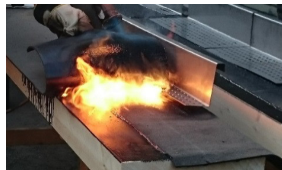
Fig. 7 Steel angle was deformed due to heating
