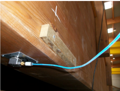
Fig. 6 Accelerometer attached under bridge girder
