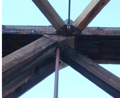
Fig. 7 Top Chord Panel Point, Through-Truss
