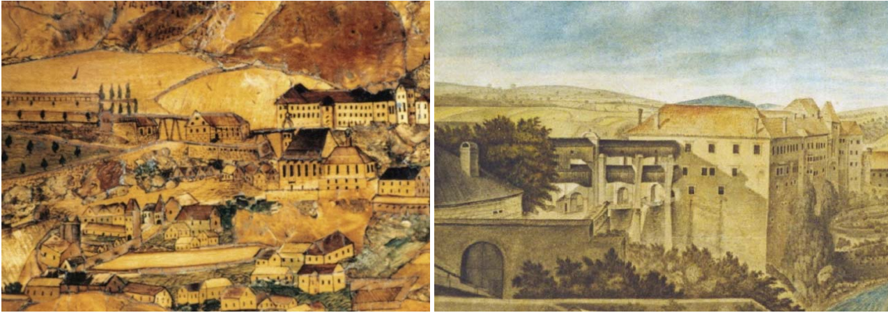
Fig. 3 Inlaid tabletop from the Krumlov Chateau collections (left) shows the situation in the early 18th century with the rear bridge leading to the garden built at the level of the theatre roof and with the simple timber bridge crossing a deep gorge by the main palace. Another view (right) from a picture dated 1743 shows that both corridors are of the same width and sheathed with planks.
