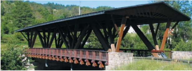
Fig. 1 Bridge on the Dore river
