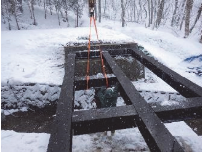
Fig. 11 Installation of main girders and cross-beams
