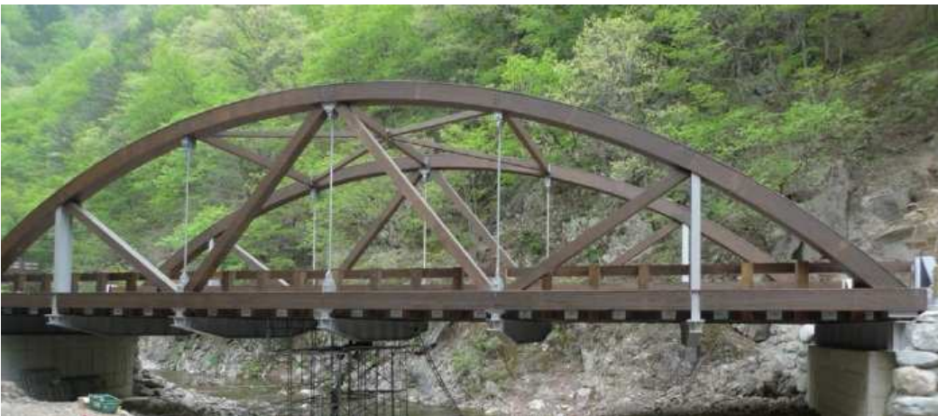
Fig. 7 Construction of Hanareum bridge
