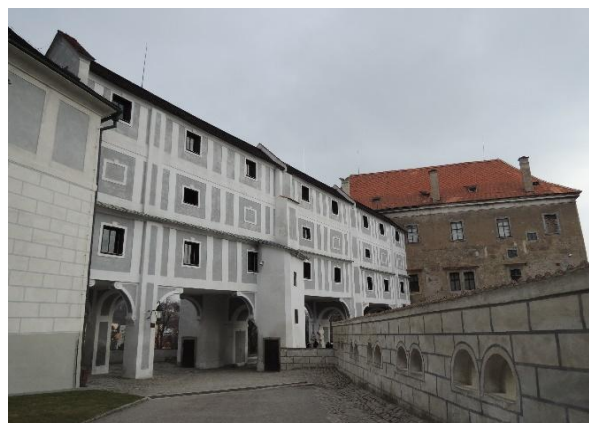
Fig. 5 Top timber part of the bridge with the cloak
