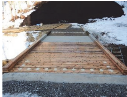
Fig. 15 Conditions prior to paving
