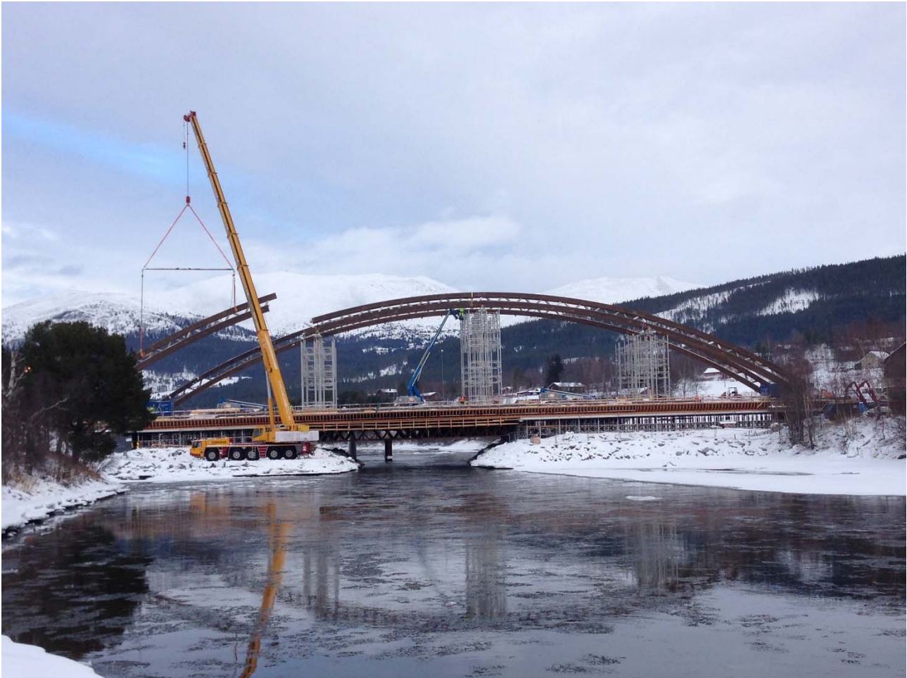
Figure 3. Steien bridge. Installation of truss arches
