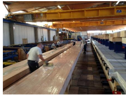
Fig. 29 Gluing of the little beams
