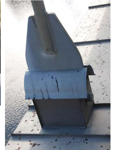
Figure 14 Hangers with welded lips covering the connection.
