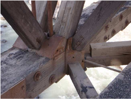
Fig. 6 Bottom Chord Panel Point, Deck Truss
