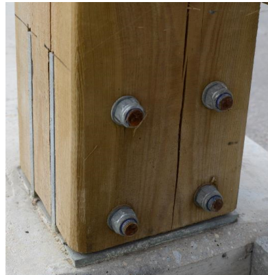
Too small washers and no steel protective coating at cut off ends.
