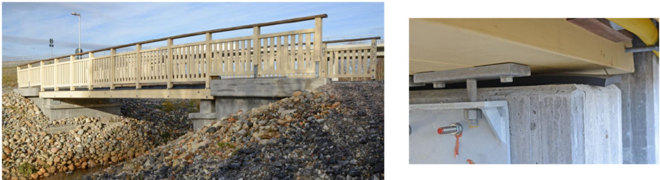
Figure 5. Left: pedestrian bridge with SLTD in Umeå, Sweden; Right: Cupping in every corner of the deck (Pousette and Fjellström 2016).
