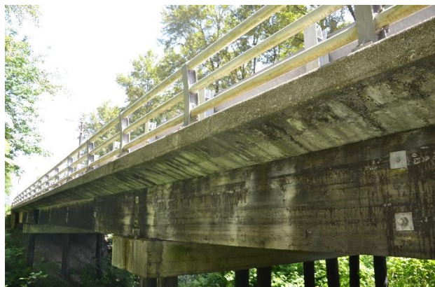
Fig. 9 Modern TCC bridge built in Singbboet Slough, Washington
