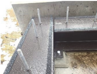
Fig. 14 Stud bolts of main girders and cross-beams
