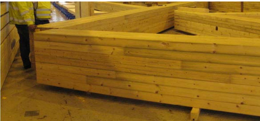
Figure 8 Example of large scale timber truss (Norsenga Bridge)
