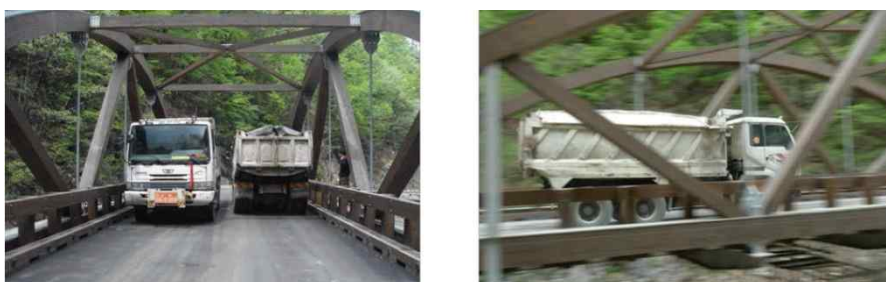
Fig. 12 Truck loading (left : static test, right : dynamic test)
