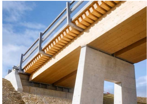
Fig. 2: Timber road bridge Horen
