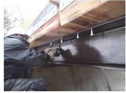
Fig. 13 Securing CLT bridge decks
