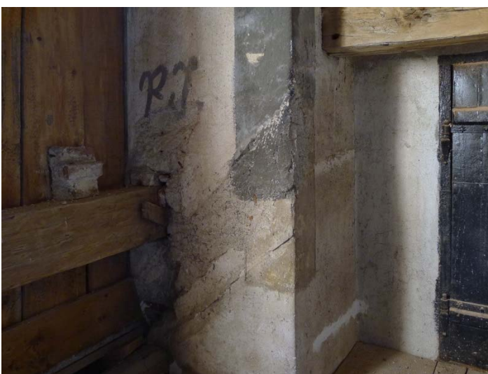
Fig. 7 Detail picture of two different colour variants giving a tectonic accent to the corners. It is clear that paint was applied before covering the roof.
