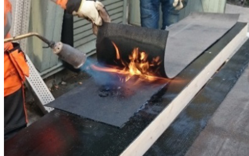
Fig. 5 Testing with splice pieces under edge strip
