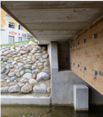
Loose bolts in girders and too small load distributing washers
