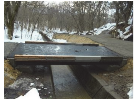
Fig. 16 Paved experimental bridge
