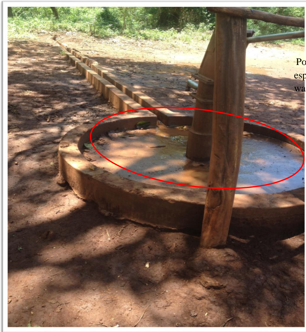
Figure 20: Budidi village borehole without a fence and under poor sanitation
