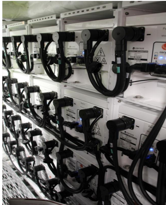
Figure 6-9: Battery pack in MS Ampere. Cells are connected in modules, sub packs and strings. The image is taken on visit to MS Ampere in October 2016.
