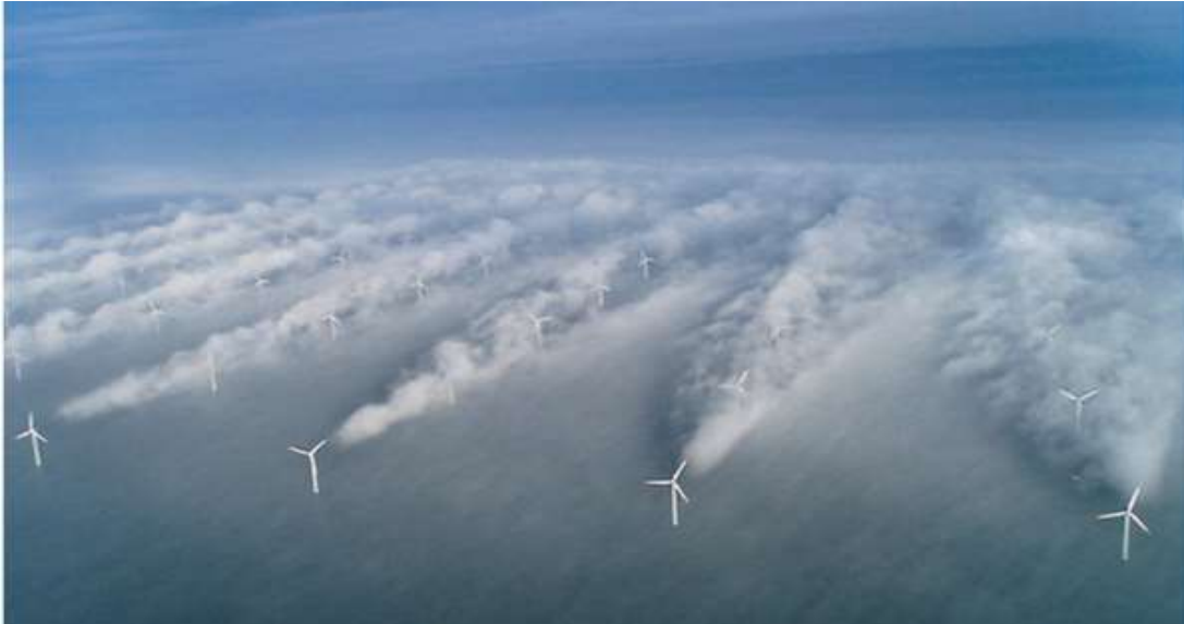
Figure 6.1. The cloud formation in the wake of the front row of wind turbines in a wind farm[45]
