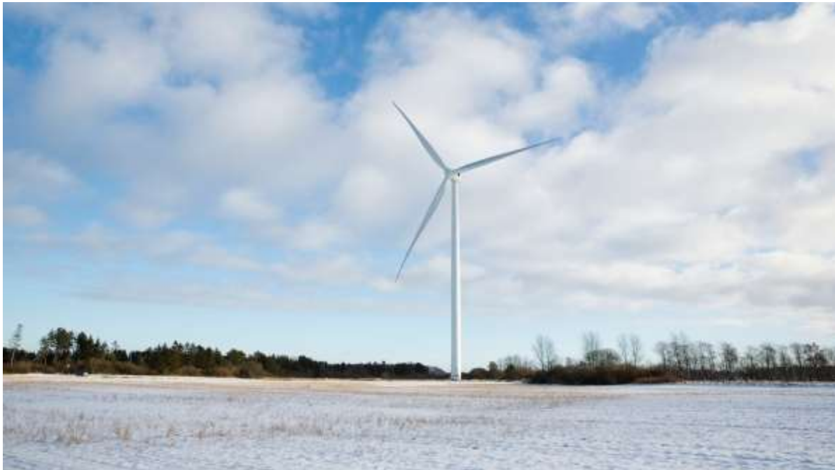
Figure C 1. Onshore Geared Wind Turbine SWT-2.3-108[48]
