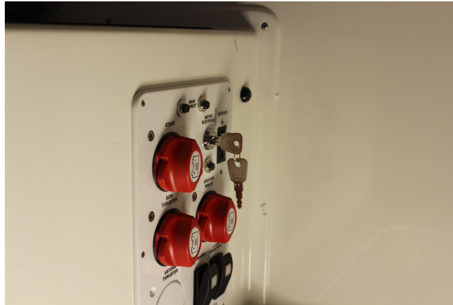
Figure 6.6 Installation of the button
