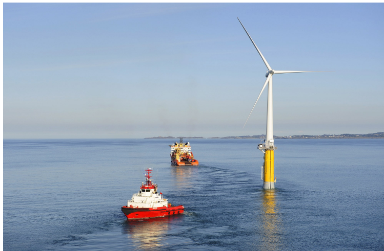
Figure 2.18: A photo from the transportation process of the Hywind turbine [2]
