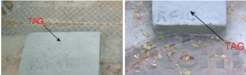
Figure 5.18: Tag under concrete at manhole.
