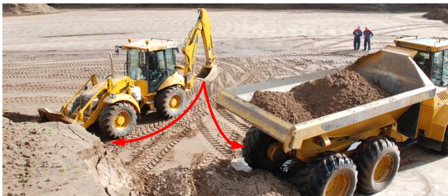
Figure 5: V-shaped motion loading a dump truck.
