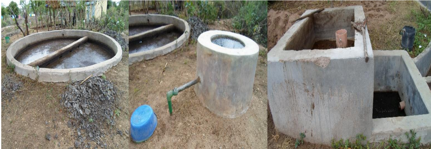
Figure 3.4 Biogas facility at Katulani SS. Output chamber is shown to the left, biogas output in the middle and slurry input with mixing device to the right
