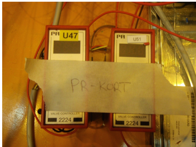
Fig 5.12 PR-card used as valve controllers for the CVG spool and the CTA valve
