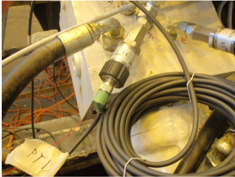
Fig 5.5 Placing of pressure transmitter PT1
