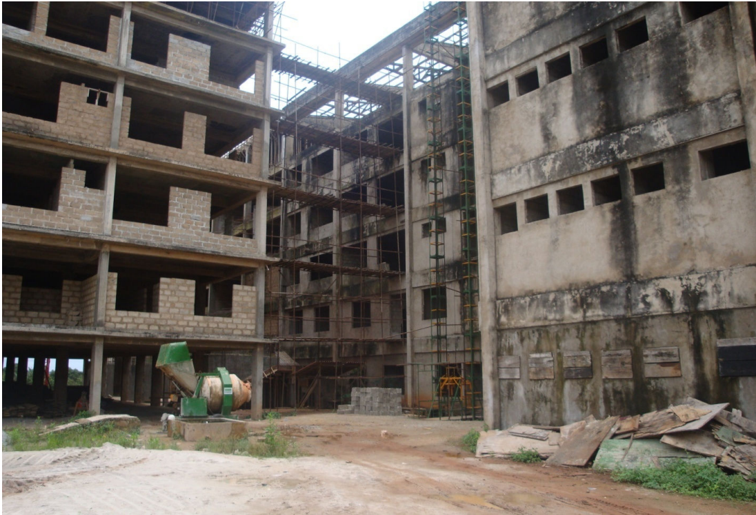
Figure 5.13: New labour ward complex under construction
