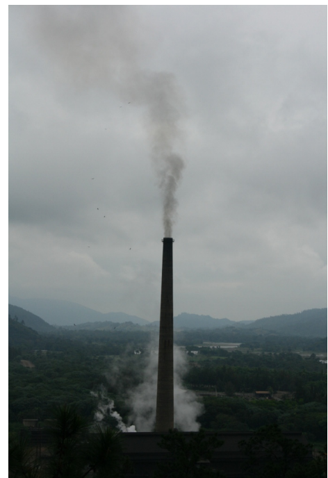
Figure 11: Falcondo Power Plant.
